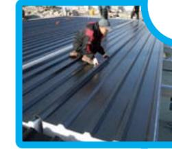
Only one-third the weight of color-coated steel, aluminum sandwich panels are easy to install.
